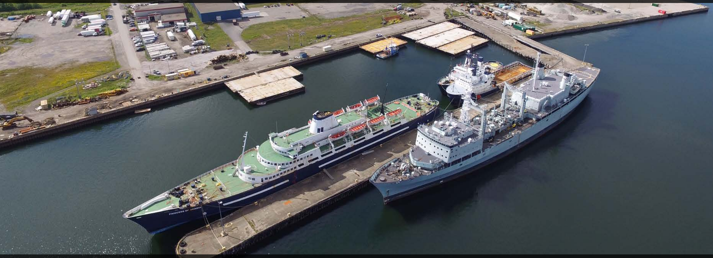
The HMCS Preserver and Princess of Acadia berthed at Sydport for recycling works
